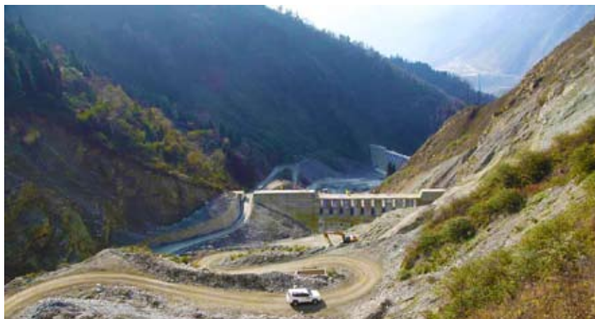
Fig. 5 Prevention measures undertaken in 2012 to reduce the debris flows hazard after the 2008 Wenchuan Earthquake (T2)
