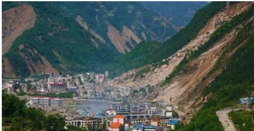
Fig. 4 Disaster in Beichuan town where landslides triggered by the Wenchuan Ms 8.0 earthquake caused thousands of deaths (T2)
