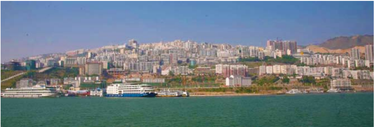
Fig .6 Relocated Wushan town built on a slope where landslides have been controlled (T3) Former town is under water.
