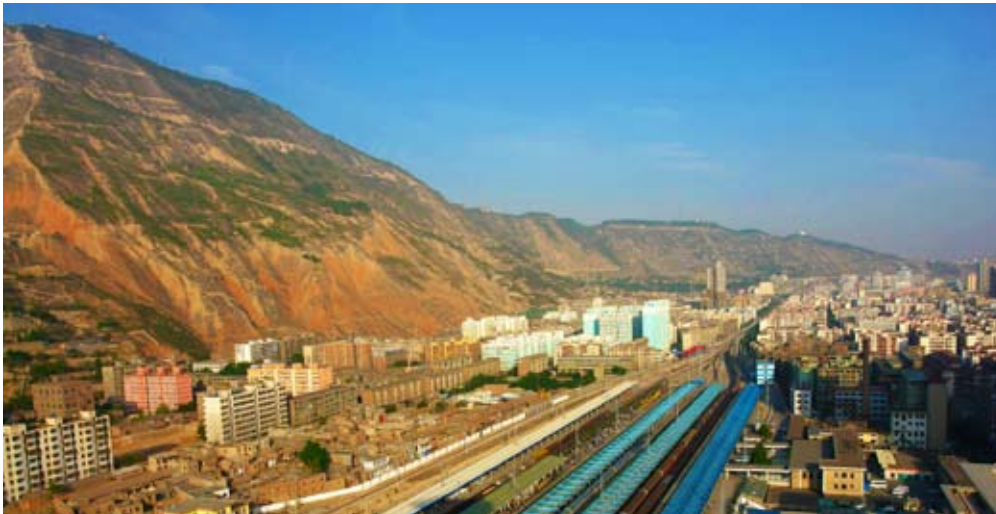
Fig. 2 The 20.56 million m 3 Gaolanshan landslide located on the southern side of Lanzhou City (T1) It consists of three sub-landslides, with multiple layers and multiple activities. The slope height is about 600 m and landslides endanger the district below it.
